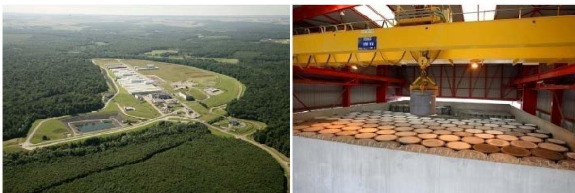
**Figure 7. Andra CSFMA disposal facility – Aerial view of the site (left) and a reinforced concrete cell in operation (right – ref ANDRA web site).**
